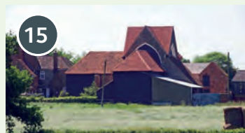
15 Latton Priory (Listed Building)
